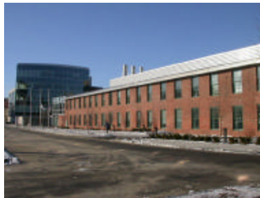
Figure 7 TKT at 28 Osborn Street
